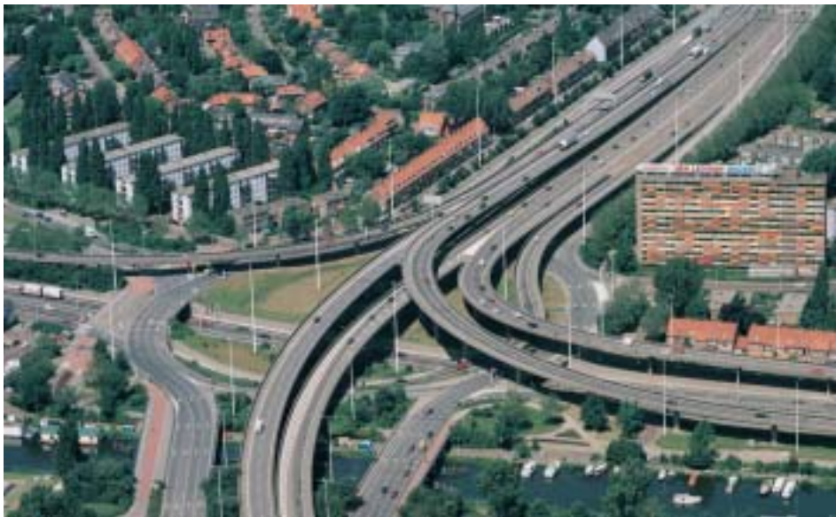
Environment and economy in the urban area: Rotterdam Overschie, residential area next to the Kleinpolderplein interchange.
