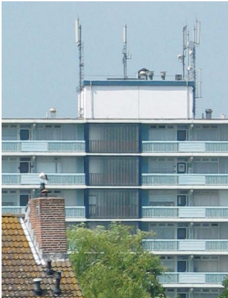
Figure 8 Example of a roof installation of GSM antennas
