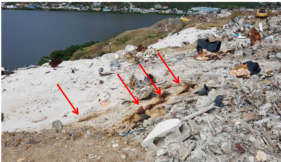
Figure 6 Smoke holes (brown/black spots marked by a red arrow) from smouldering fires inside the landfill.
