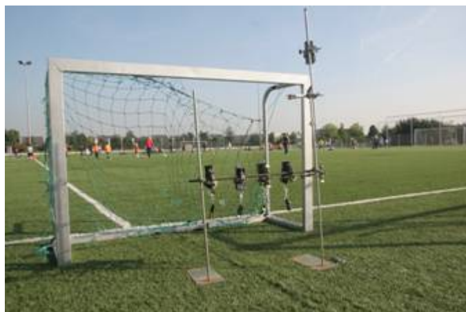
Photograph 6 Five pumps at Rijkerswoerd
