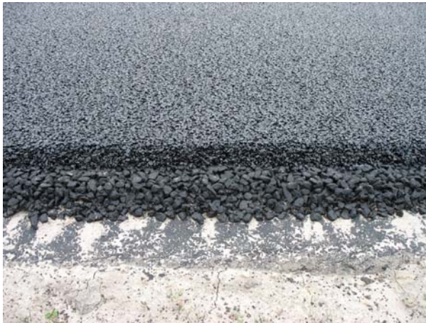
Figure 2 Double Layer Porous Asphalt (DLPA) at the A2 motorway near Breukelen.
