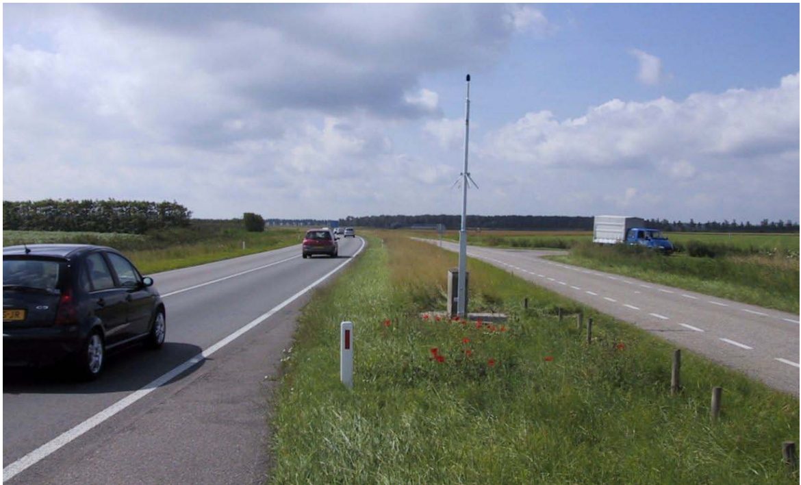
RIVM monitoring site at N256 motorway (Noord-Beveland).
